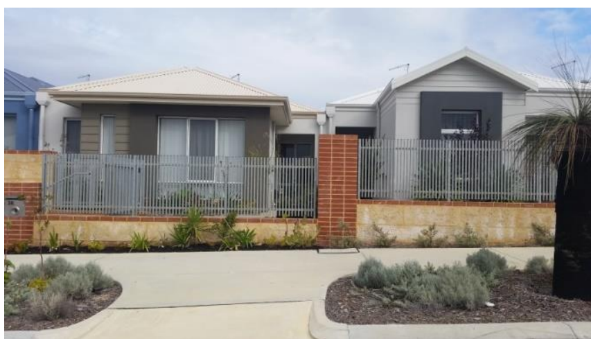
Image 4: Cohesive and consistent front boundary fencing installed by the developer
