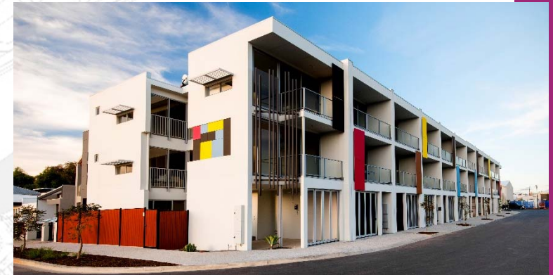
Clearly defined ground floors enhance public realm, with upper levels providing opportunities for passive surveillance of the public realm.
