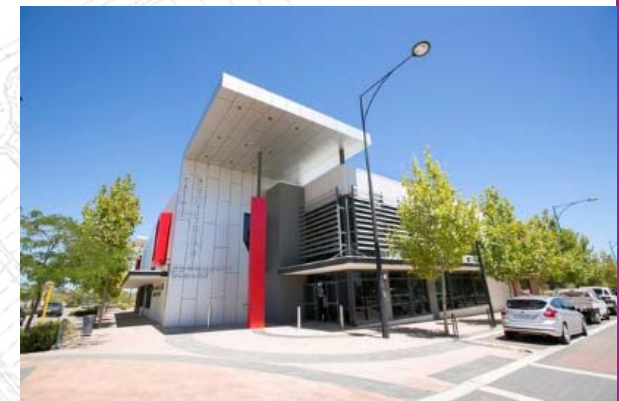
Windows, openings and balconies address the street to encourage active use of this zone.
