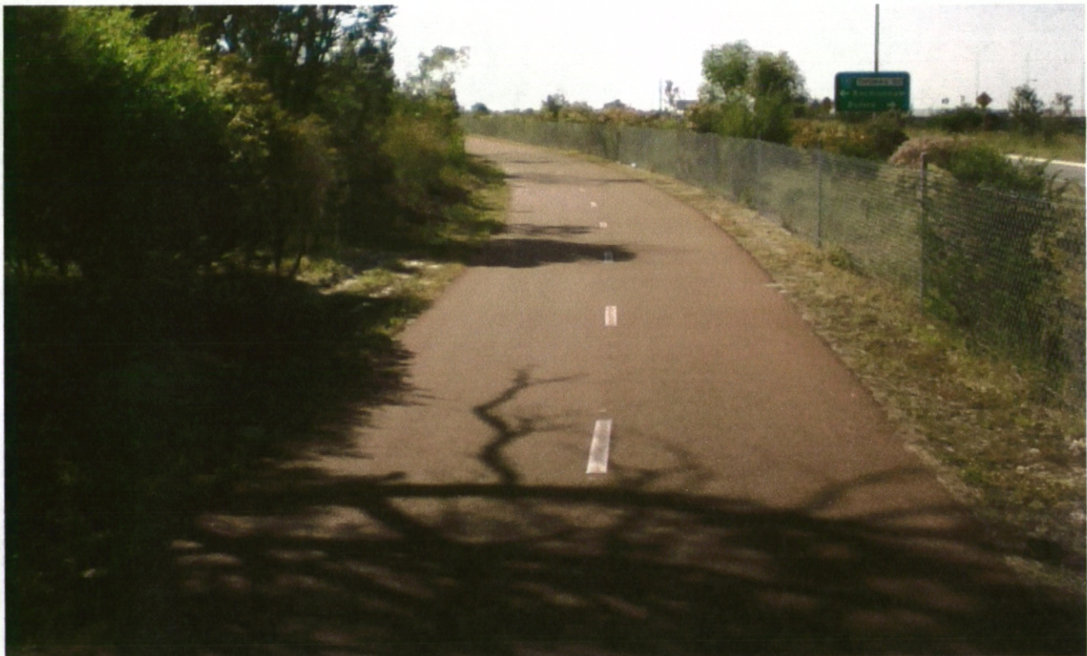
Plate 3 Adjoining Kwinana Freeway dual Use Path Looking North
