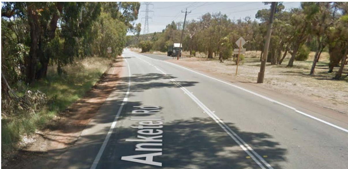
Figure 7-5 Sealed Shoulders on Anketell Road
