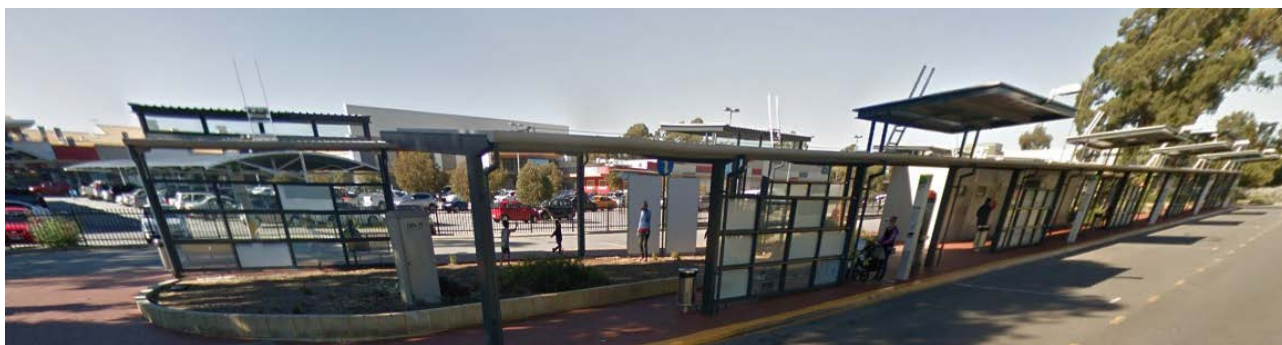
Figure 3-1 Kwinana Bus Station
