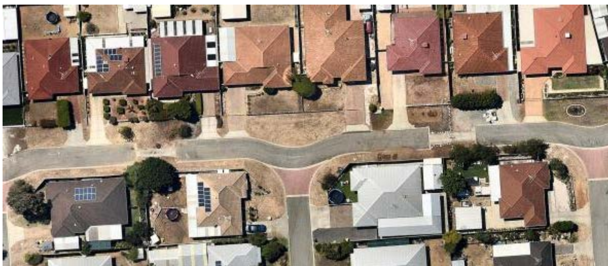
Figure 8-2 Residential Development Without Footpaths, Wellard
