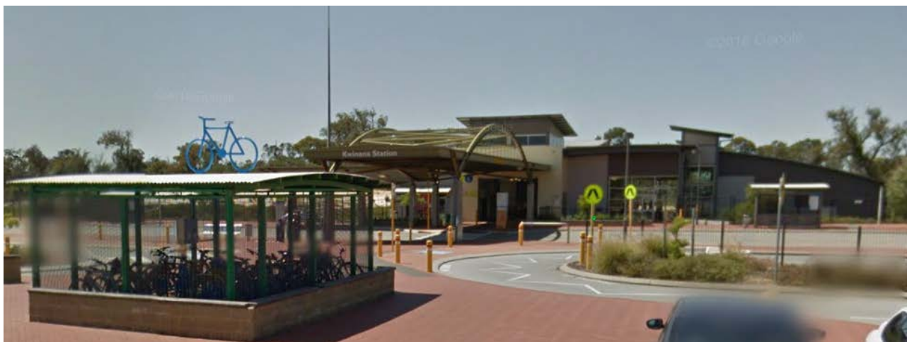
Figure 9-5 Bike Shelter at Kwinana Train Station
