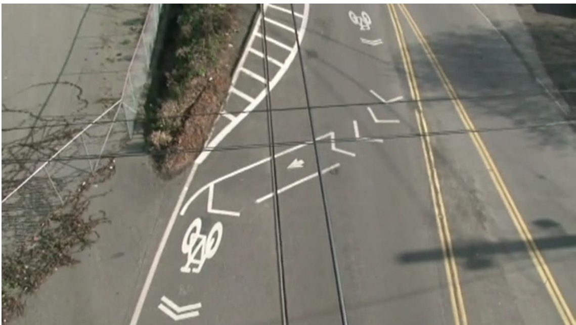
Figure 9.10: Rail angled crossing treatment example
