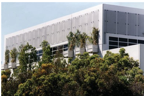
'Green screens', in fencing and on building façades and courtyard walls, can significantly reduce heat loads and improve air quality
