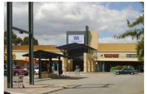
The existing Kwinana Hub shopping centre
