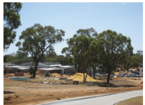
The new high school under construction in the Education Precinct
