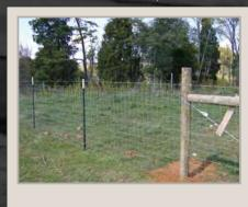
CONSERVATION FENCE 1.2m high reserve fence with ringlock mesh, top wire and galvanised steel picket posts to core edge. 3.5m wide access gates with treated timber posts every 400m.
